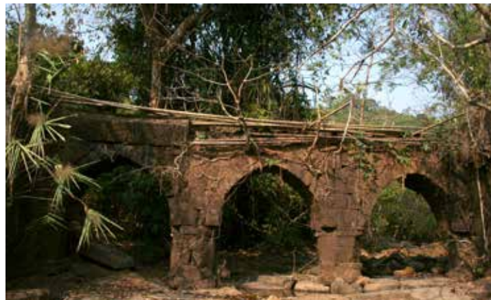
Arched stone bridge built during the reign of Jaintia Kings near Syndai in West Jaintia Hills.
